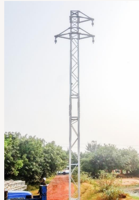
Rebar lacing pole
