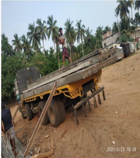
Loading of Material
