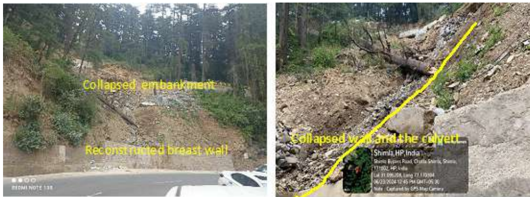
Image 4.14 - The central part between NH5 and the first, middle local road prominently damaged due to the excessive flow of rainwater over the slope.
