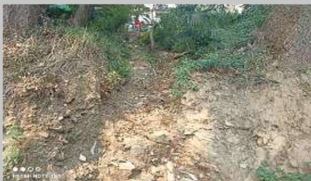
Image 4.18 - Unlined drainage from higher slope opening persistently onto it
