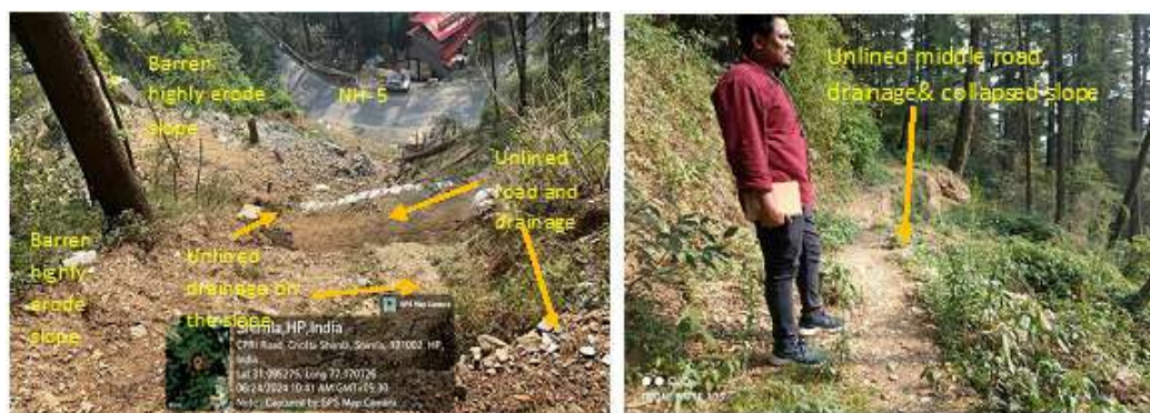
Image 4-15. A top view with three roads: barren slope, unlined drainage, and collapsed slope
