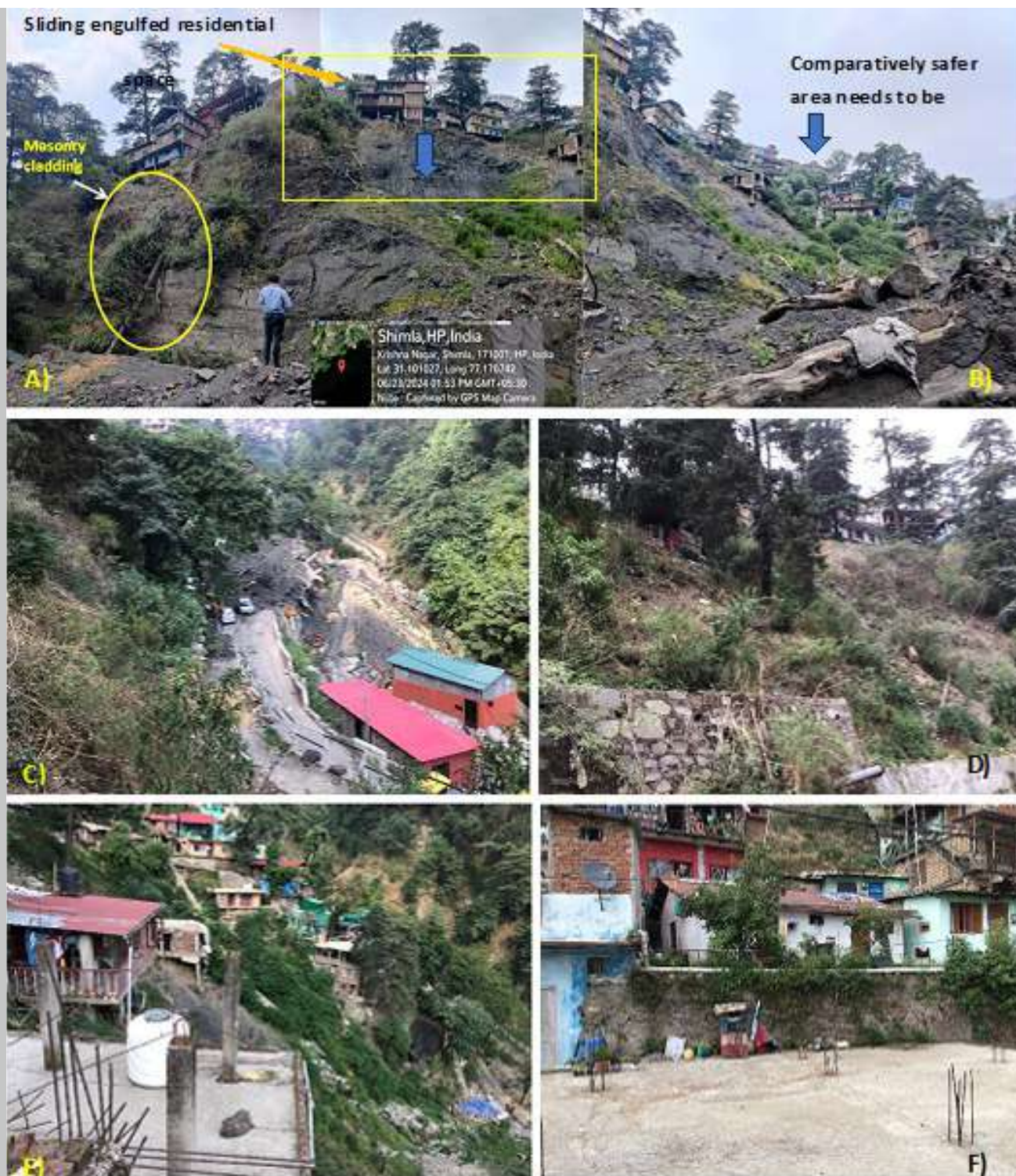
Image 4.11 - (A-B) Landslide view, (C) Vulnerable houses and settlements, (D) Lower portion of the landslide exposed to infiltration, and (E-F) Buildings closer to the landslide scarp
