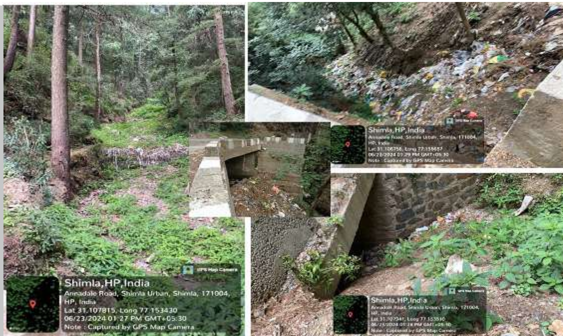
Image 4.44 - Streams found dumped with waste material, culverts choked, and drains half full
