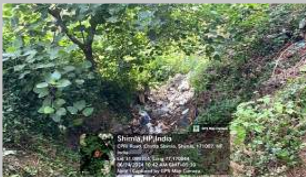
Image 4.17 - Dumping of slope drainage and unlined temporary drainage opening directly on the slope
