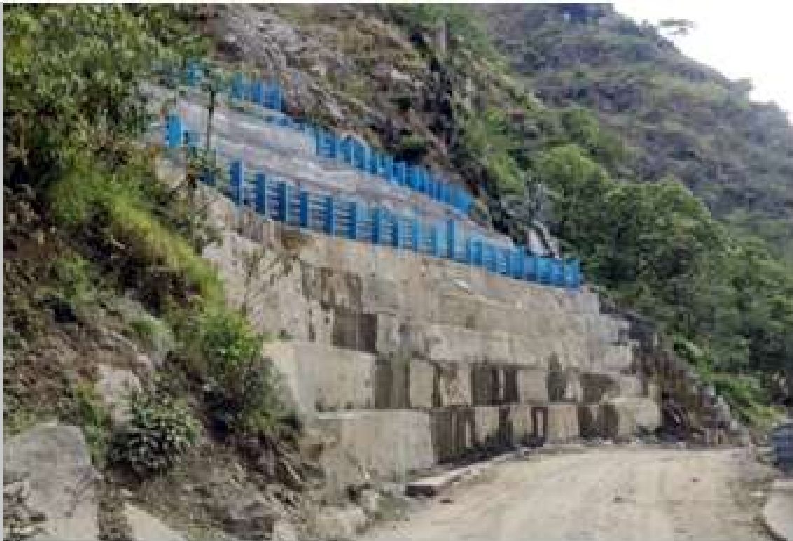
Image 4.9 - Typical photograph of slope stabilization with CC cladding and fencing
