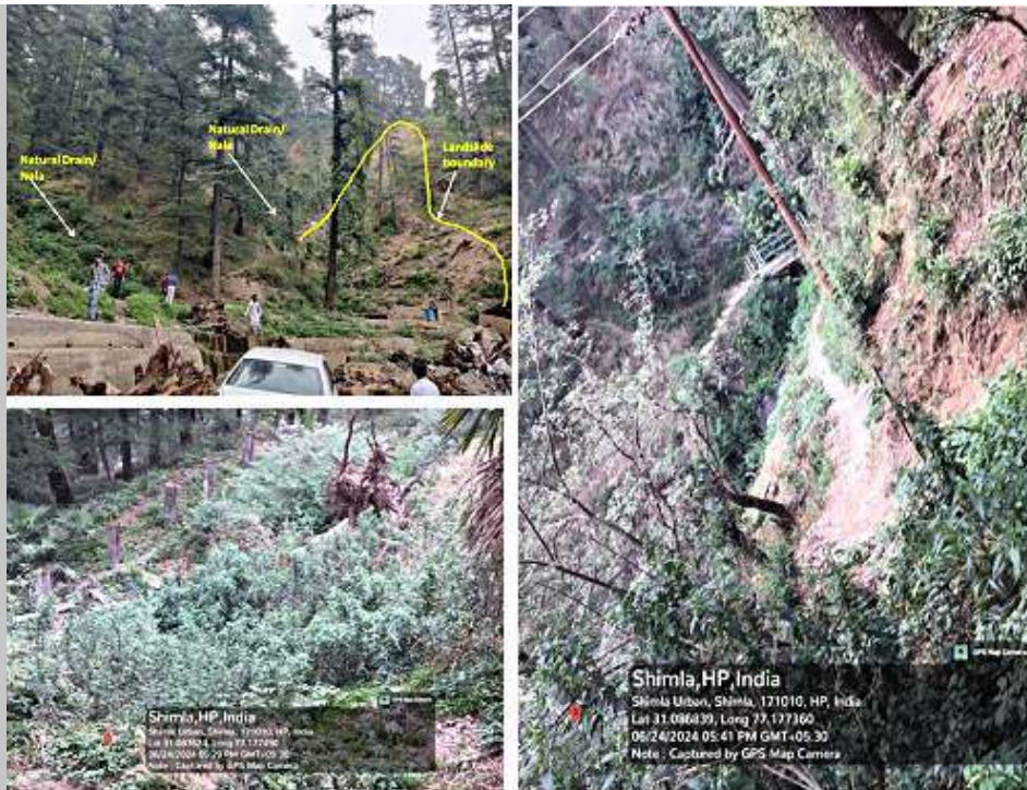
Image 4.27 - Streamside slope failure, subsidence, intensive erosion, and slope failure
