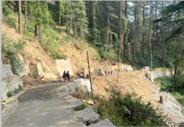
Image 4.16 - Middle road leading to habitation severely damaged, roadside slope, reattaining wall, and slope failure
