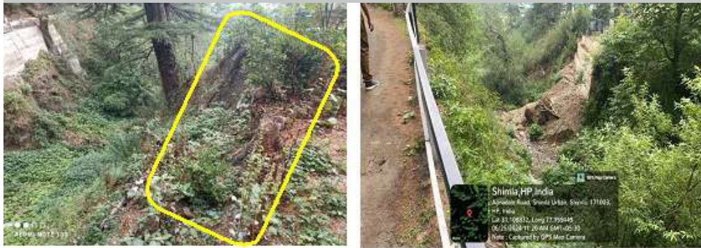
Image 4.34 - The park which divides the streams is severely eroded, subsided, and cracked
