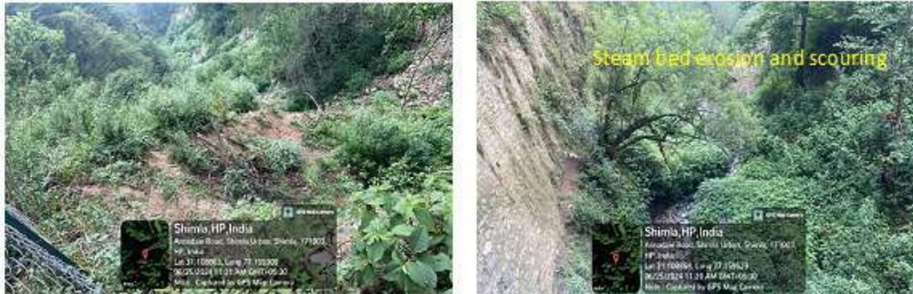
Image 4.36 - The park which divides the streams is severely eroded, subsided, and cracked
