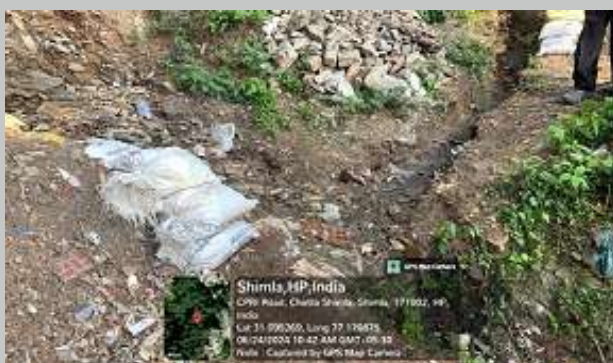
Image 4.18 - Unlined drainage from higher slope opening persistently onto it
