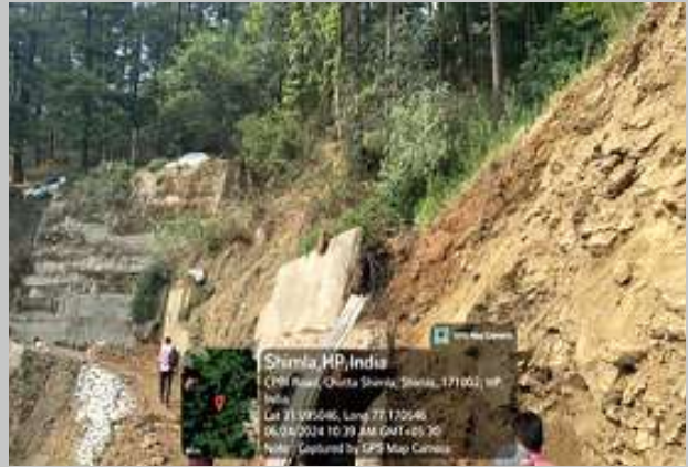
Image 4.16 - Middle road leading to habitation severely damaged, roadside slope, reattaining wall, and slope failure
