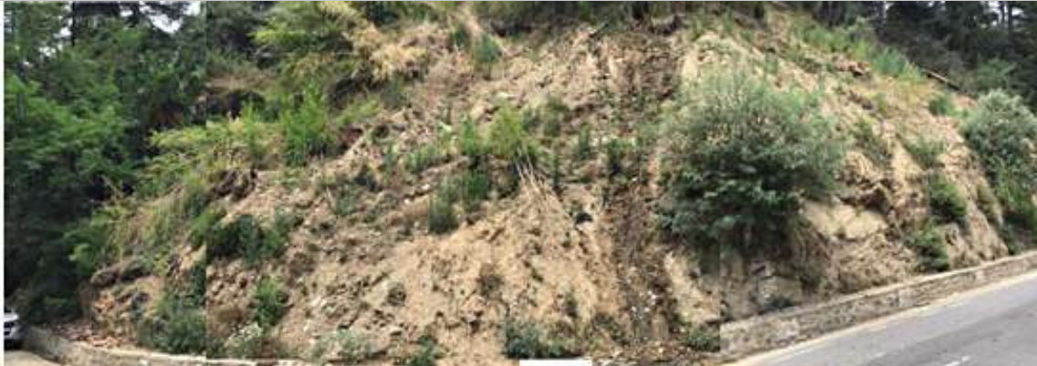
Image4.20 - Roadside landslides in thick colluvium deposits are mainly attributed to inadequate drainage and protection measures
