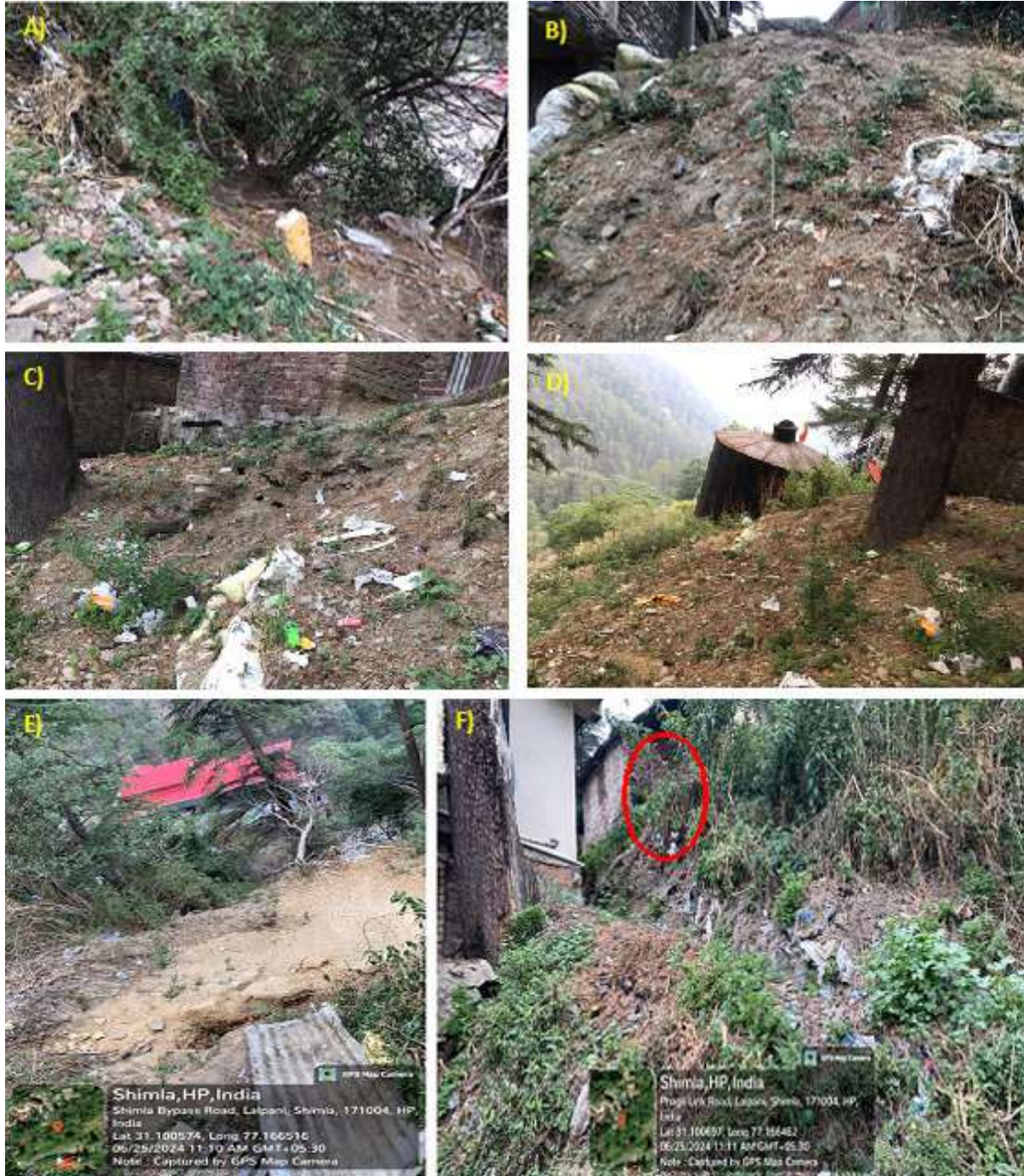
Image4.8- Major activities observed in the landslide area. (A-B) Mismanaged slope with domestic dumping waste, (C-D) Cracked and subsided land closer to the landslide scarp, and sandbags can be seen stacked to prevent subsidence/sliding, (E) Unauthorized foundation being dug for construction of retaining wall on the top of the slope, and (F) Temporary drain made opens directly on the slope.
