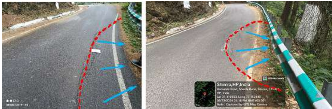
Image 4.39 - Subsidence and cracks on the road surface Note: Circular cracks were noticed towards the tree
