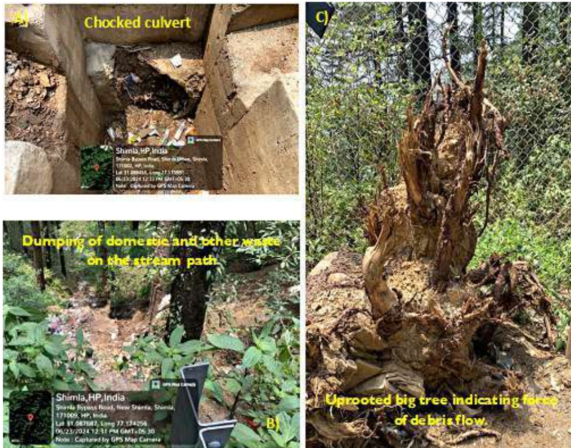
Image 4.23 - Activities observed along NH5 and downslope. (A) Choked culvert, (B) Dumping of wastes, and (C) Uprooted trees
