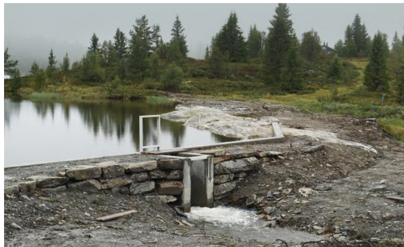
The old stone masonry dam after modifications completed
