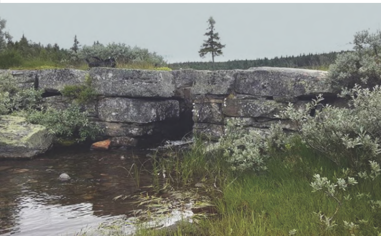
The old stone masonry dam from 1870 at Lake Svintjønna before revitalization
