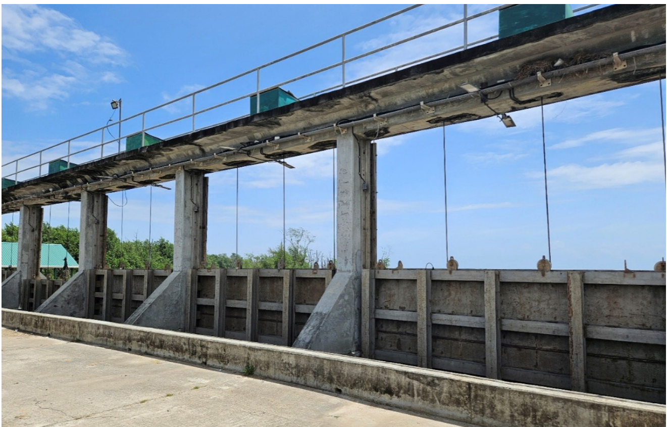
Figure 17. The Hope Canal outfall sluice
