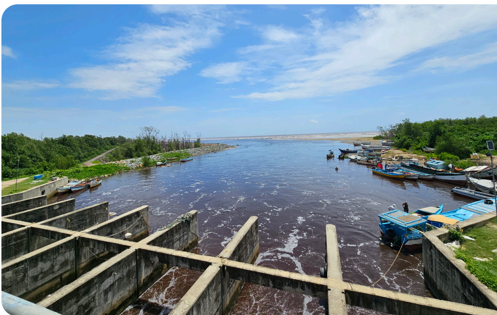
Hope Canal outward flow into the North Atlantic Ocean, built after the 2005 floods to release excess water from the East Demerara Water Conservancy (EDWC) into the Atlantic Ocean via an 8-door sluice.
