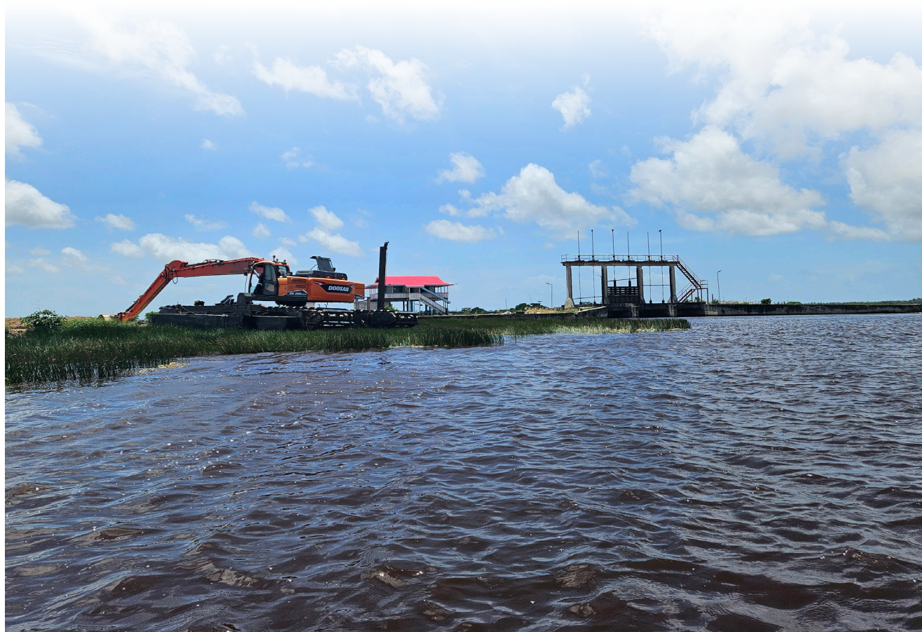
An amphibious dredging machine positioned along the edge of the waterbody, carrying out rehabilitation and dredging activities within the East Demerara Water Conservancy.
