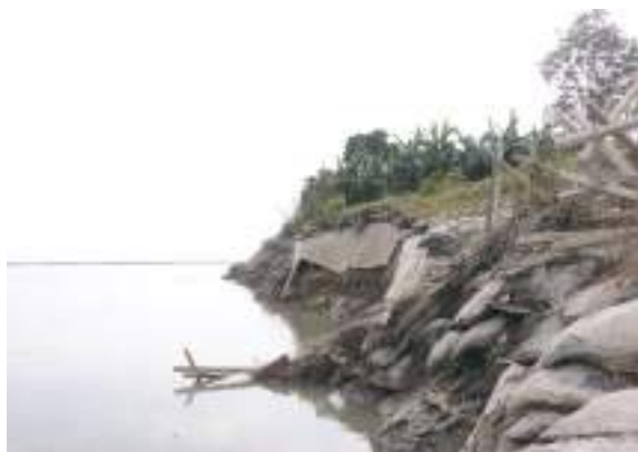
Figure 15.(a) Destroyed sandbags
